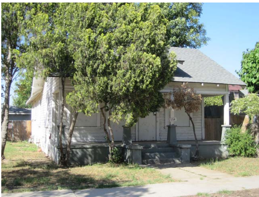
3343-59 4 th Street, View from 4 th Street looking north (May 3, 2010)
