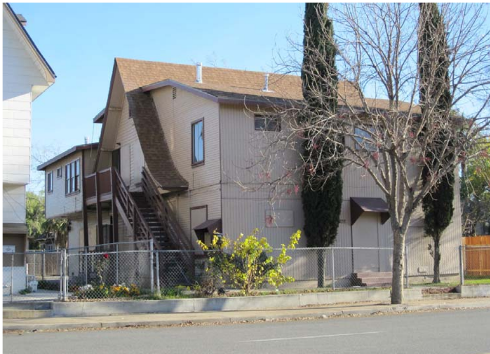
3478 Lime Street, View of Lime Street façade looking west (January 5, 2010)
