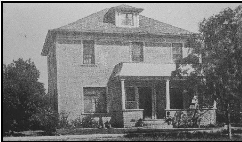
460 Lime Street (Source: Riverside Fire Dept, Souvenir of the City of Riverside , 1906)
