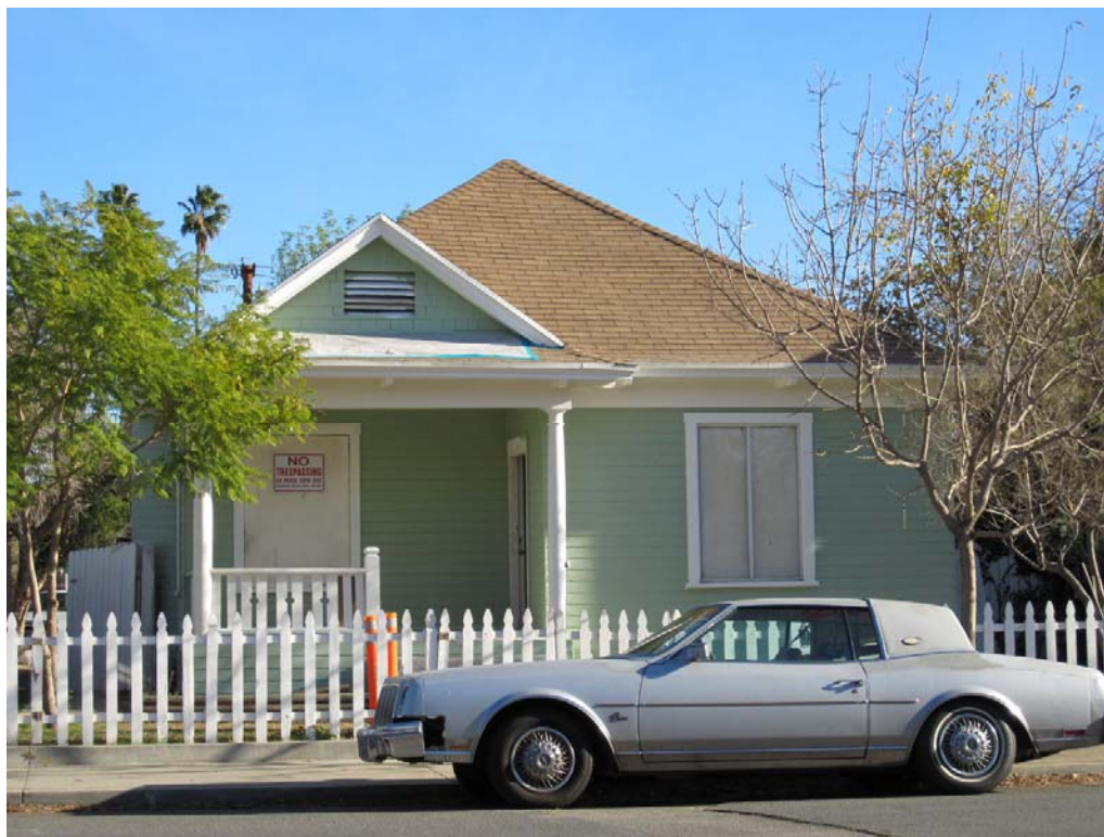
3426 Lime Street, View from Lime Street looking west (May 3, 2010)
