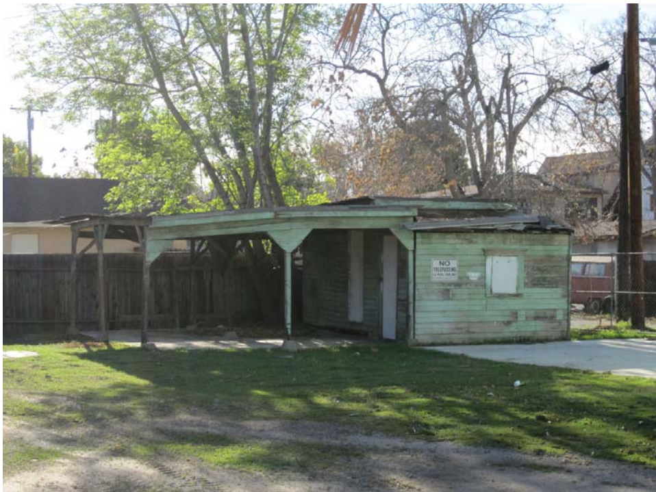
3344-46 4 th Street, View of carport/tool shed looking southwest (May 3, 2010)
