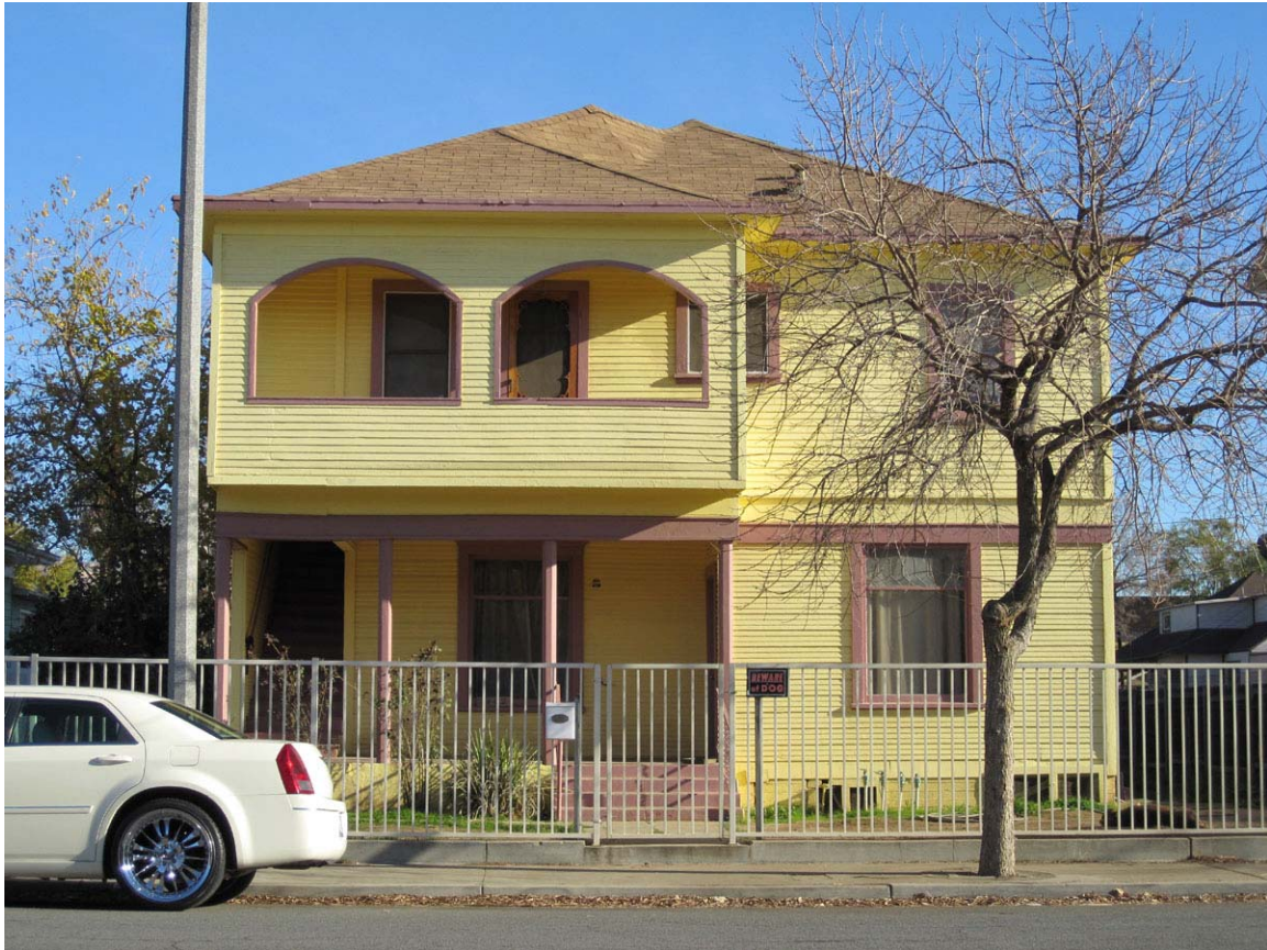
3442 Lime Street, View from Lime Street looking west (May 3, 2010)
