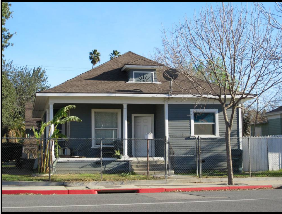
3390 4 th Street/3410 Lime Street (Source: Page & Turnbull, January 5, 2010)
