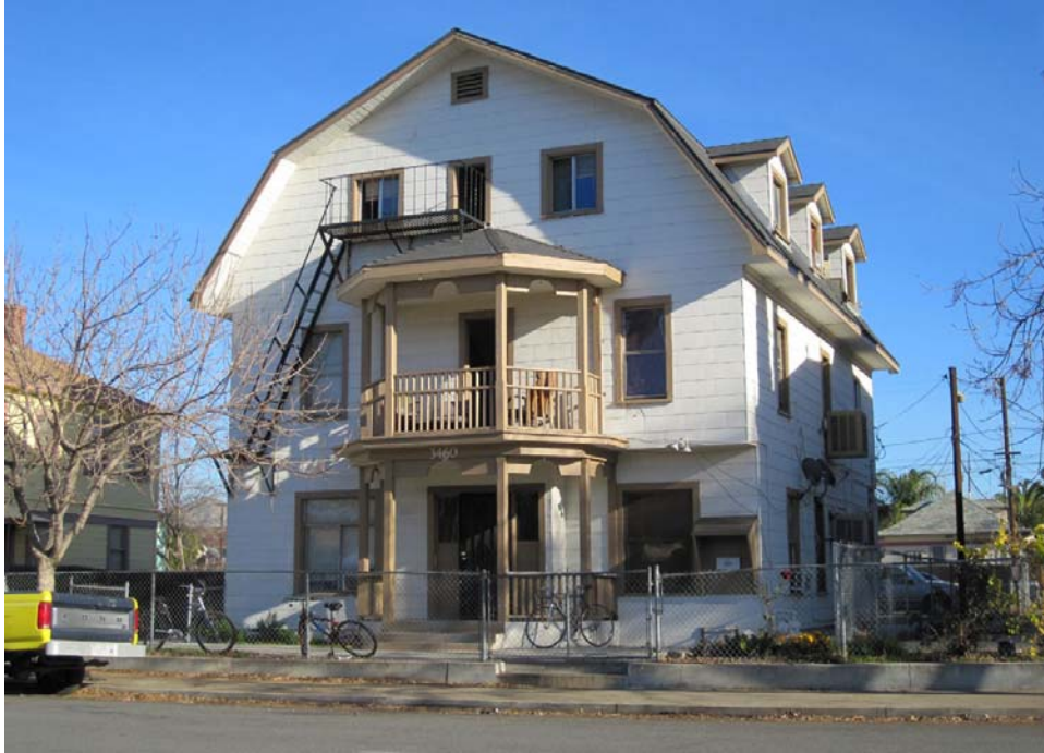
3460 Lime Street, View from Lime Street looking west (May 3, 2010)
