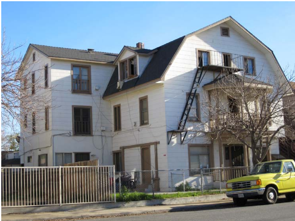
3460 Lime Street, View from Lime Street looking northwest (May 3, 2010)
