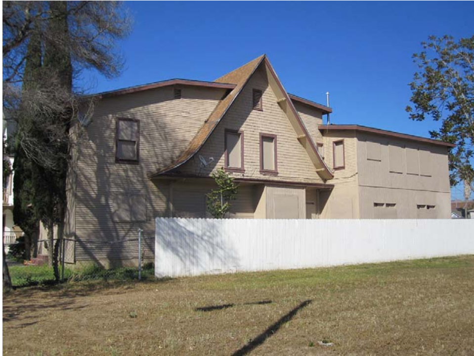
3478 Lime Street, View looking south (May 3, 2010)
