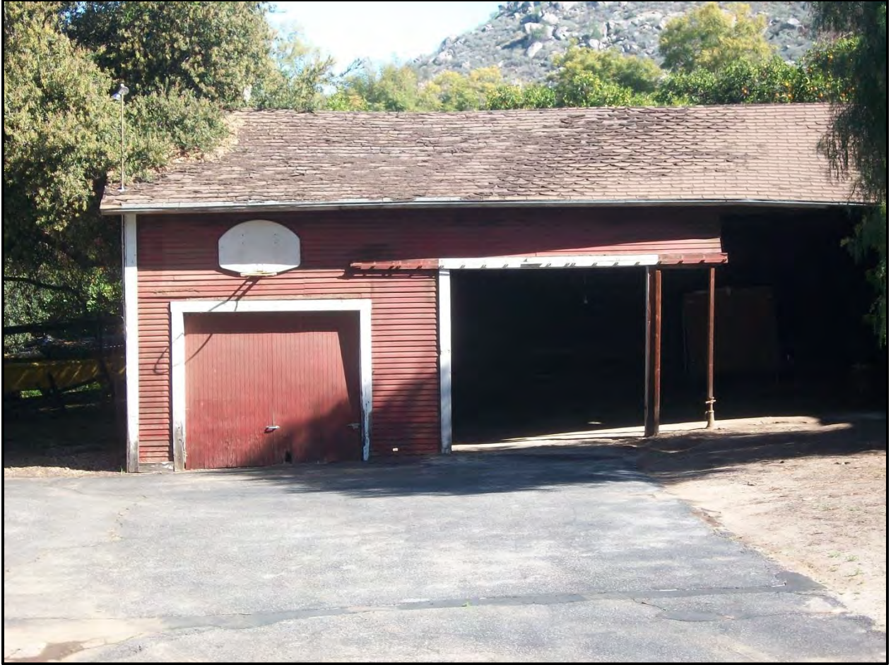
Figure 18. South Elevation of the Merriman Garage/Barn (facing North/Northeast).
