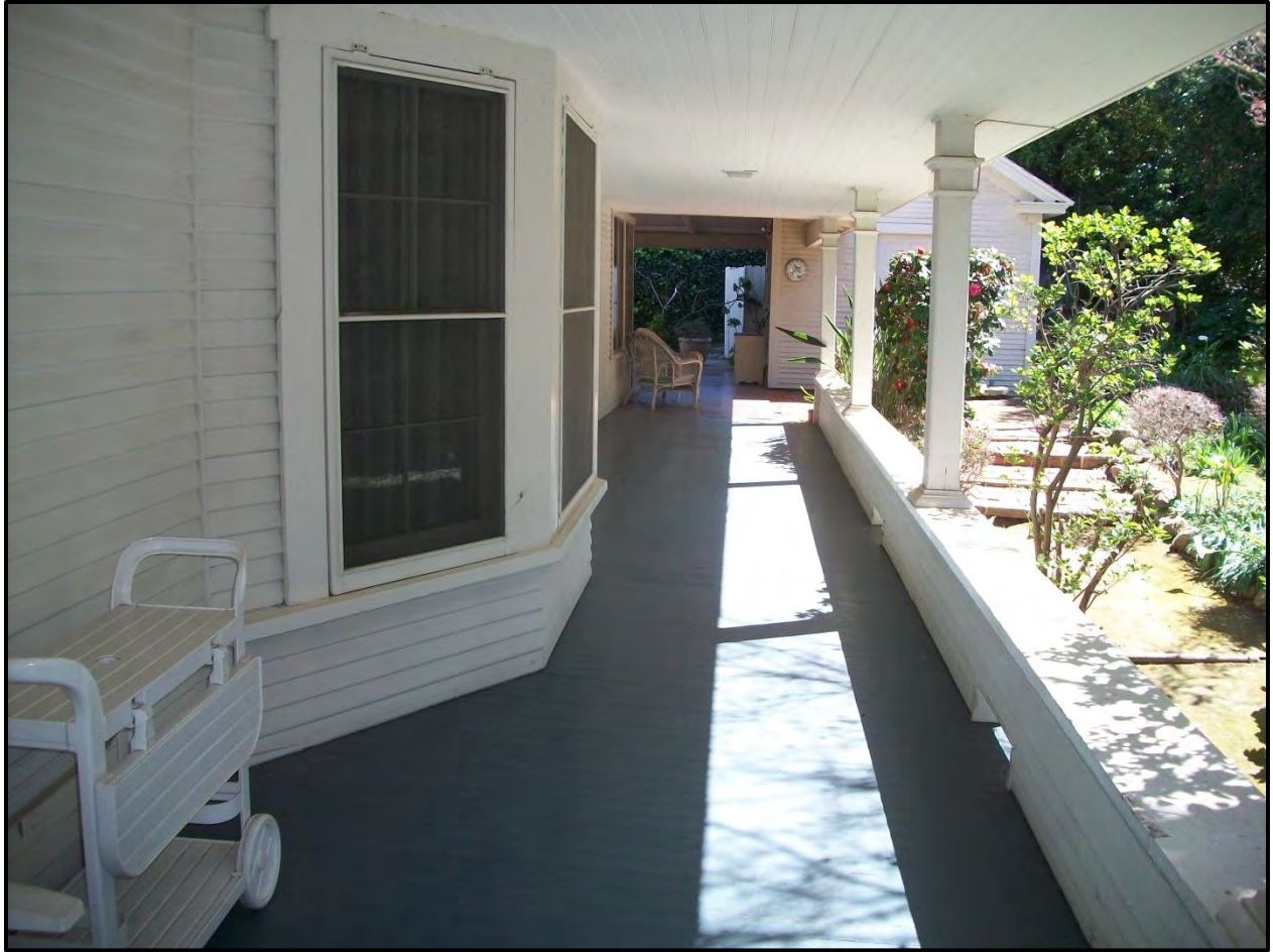
Figure 13. Overview of South Elevation Porch of the Walton Residence from the Southwestern Corner of the House (facing East).
