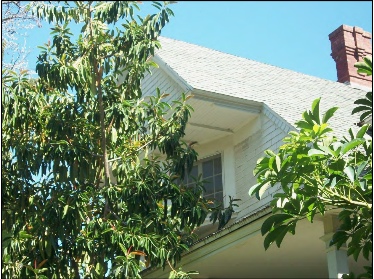
Figure 15. Second Story Overhanging Roofline on West Elevation (Northeast).
