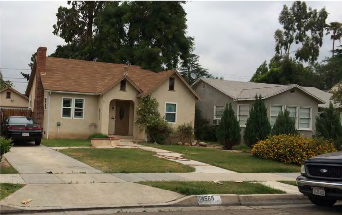
Home with Vinyl Windows on Left; Home with Original Windows on Right
