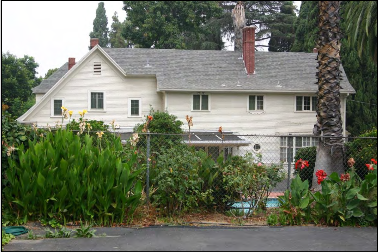
Figure 16. East Elevation of the Walton/Merriman Residence (facing West).
