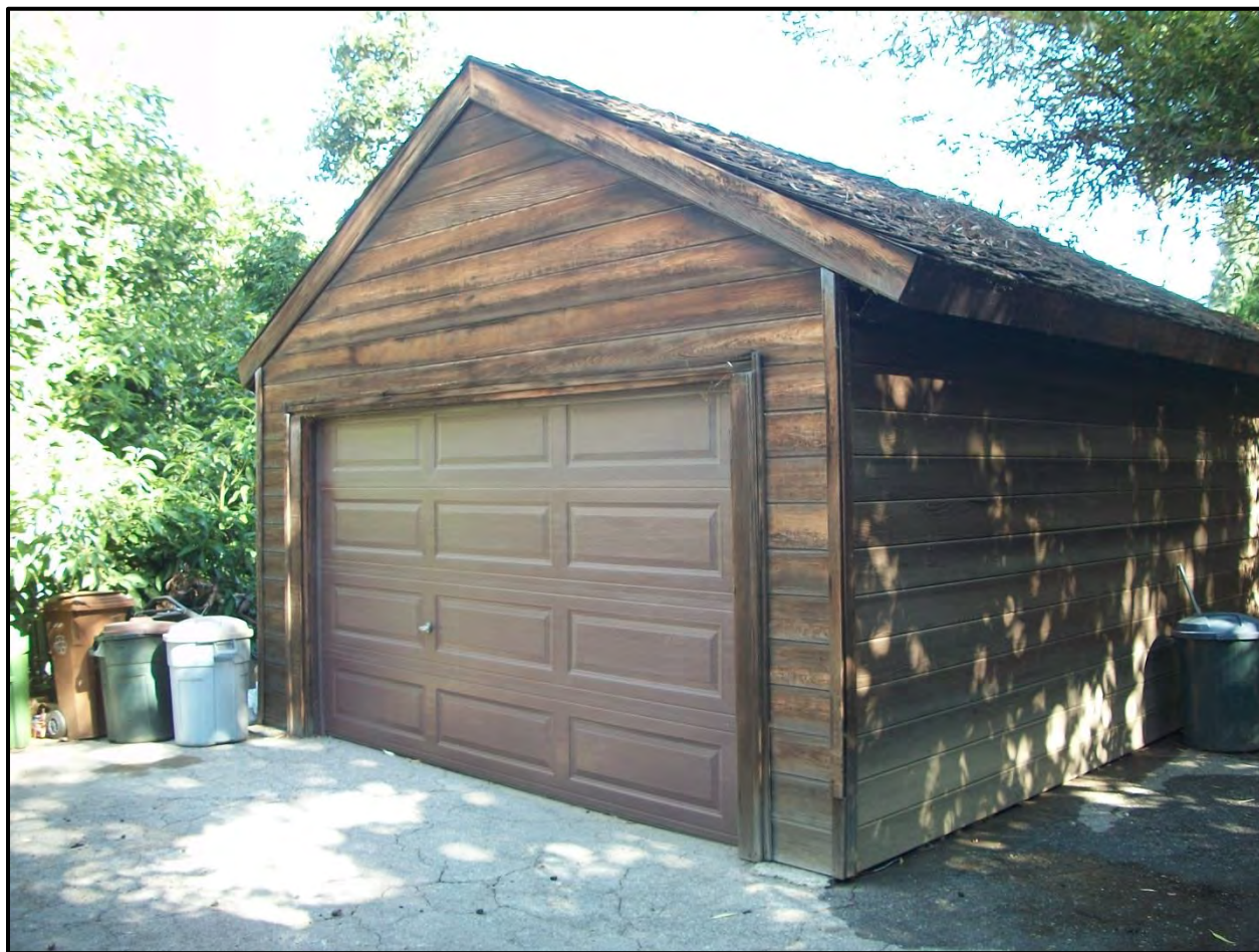
Figure 25. The Lawson 1975 Garage (facing Northwest).
