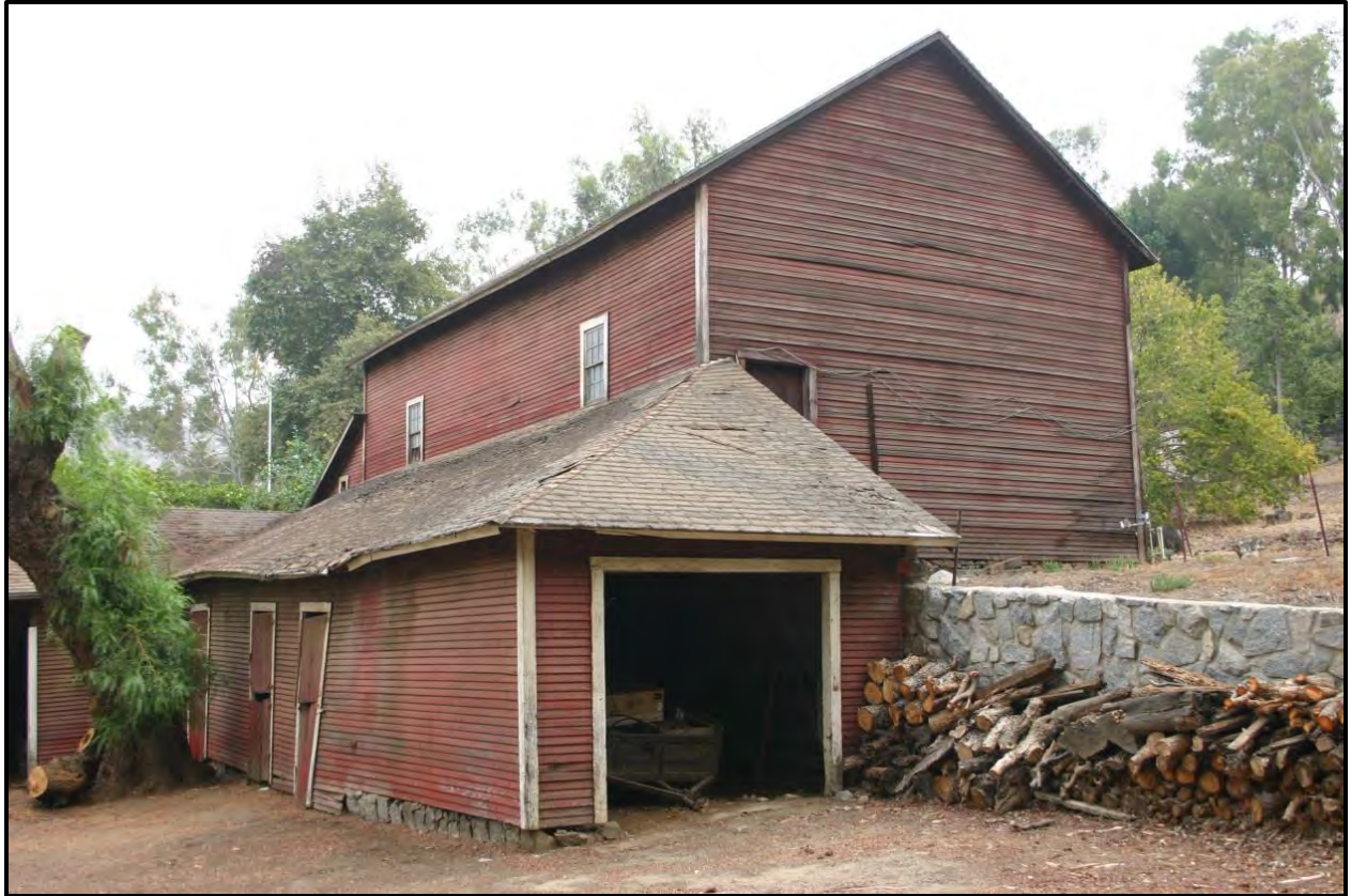
Figure 17. Main Barn and Stable at the Walton/Merriman Property (facing Northeast).
