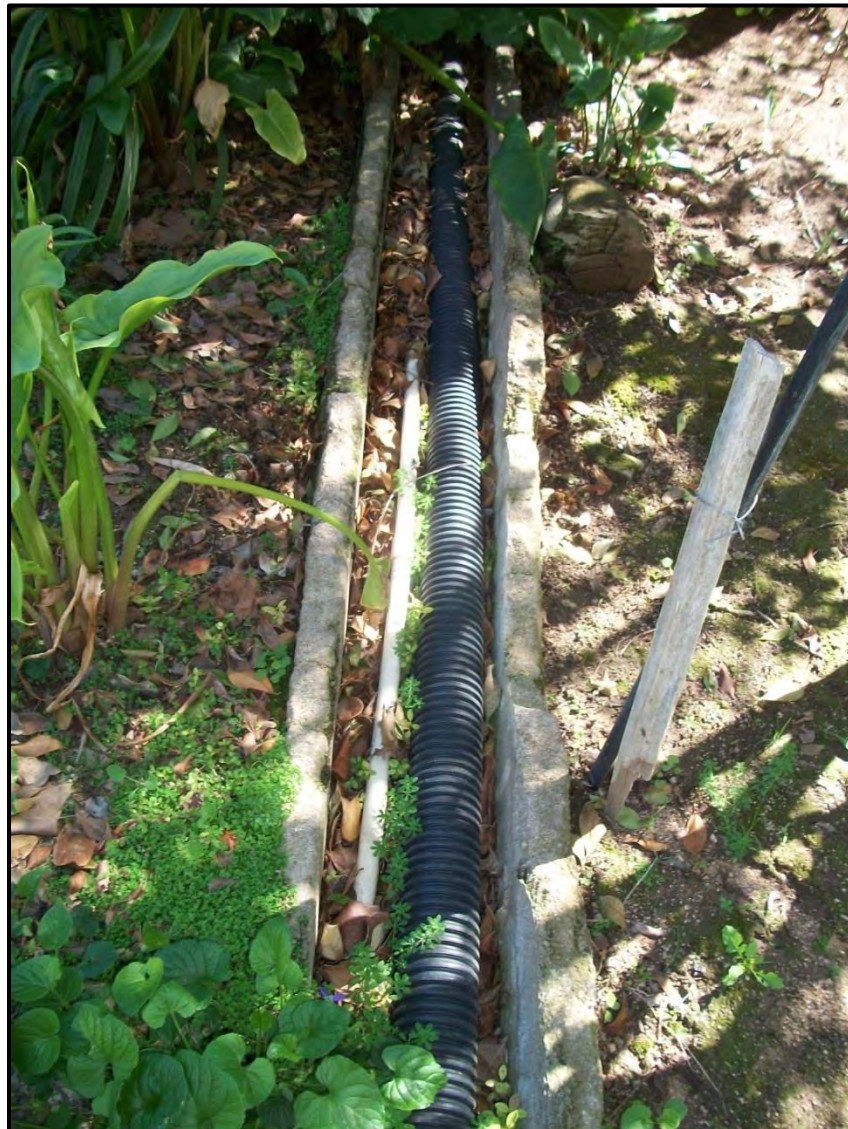
Figure 20. Irrigation Trough Identified West/Northwest of the Walton Reservoir.
