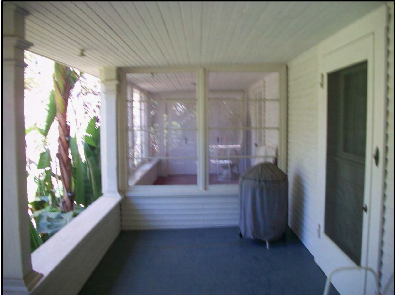
Figure 14. View of the West Elevation of the Walton Residence from the Southwestern Corner of the Wrap-Around Porch (facing North).
