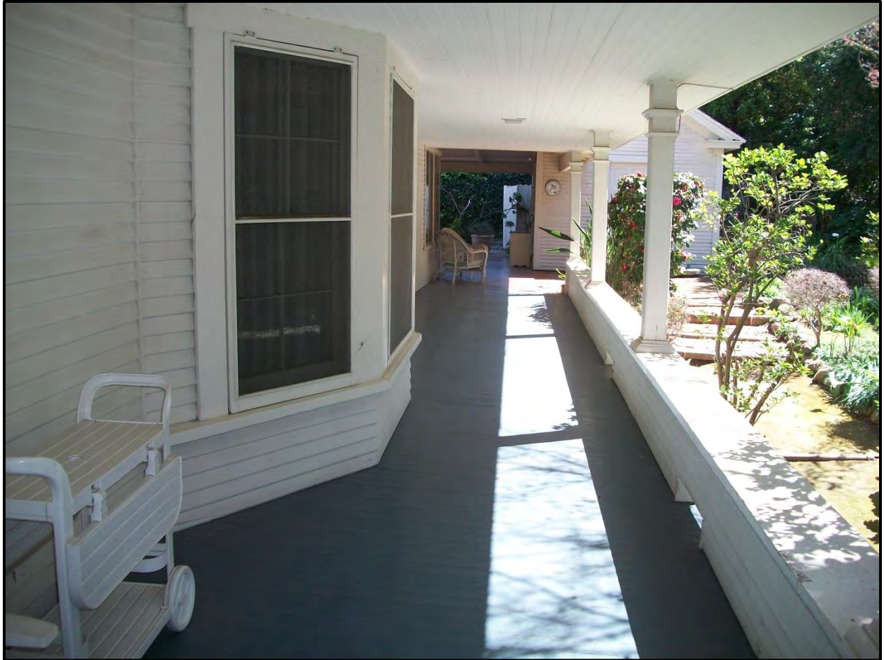
Figure 13. Overview of South Elevation Porch of the Walton Residence from the Southwestern Corner of the House (facing East).
