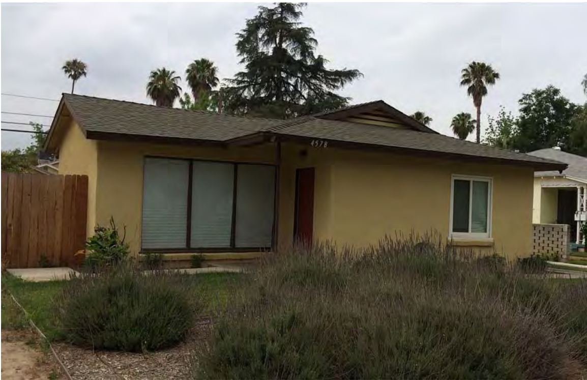
Adjacent Site - 4578 Sunnyside Dr (Non-contributor)
