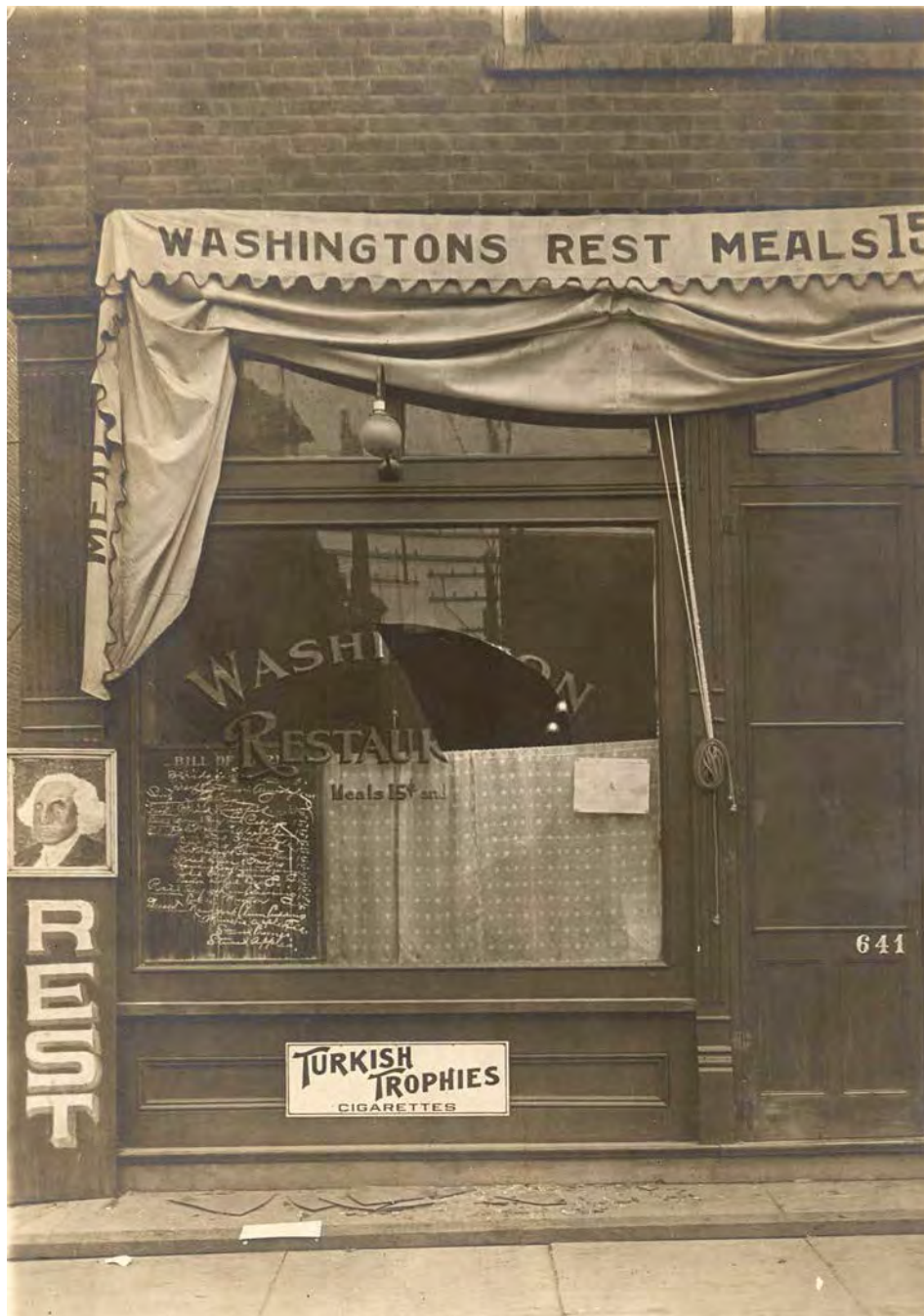
3. Washington Restaurant with Broken Window, 1913 Courtesy Riverside Metropolitan Museum
