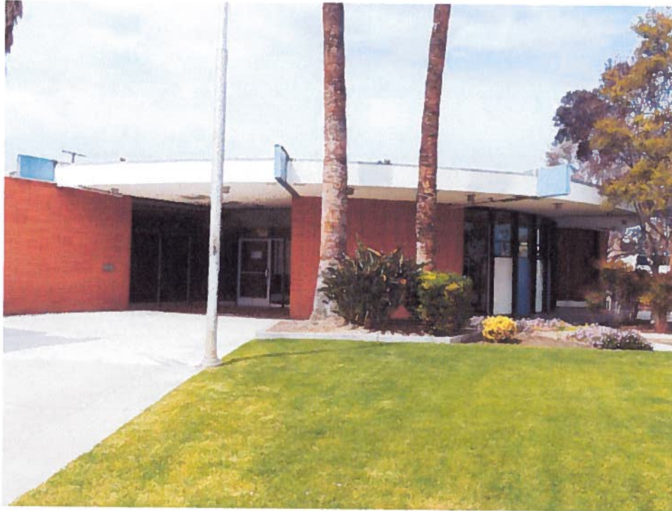
Detail of Entry, looking North (March 2013)
