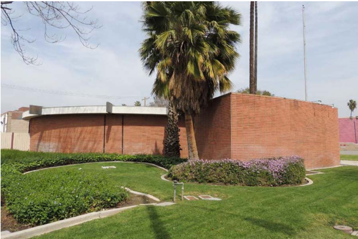
View of West Facade looking East
