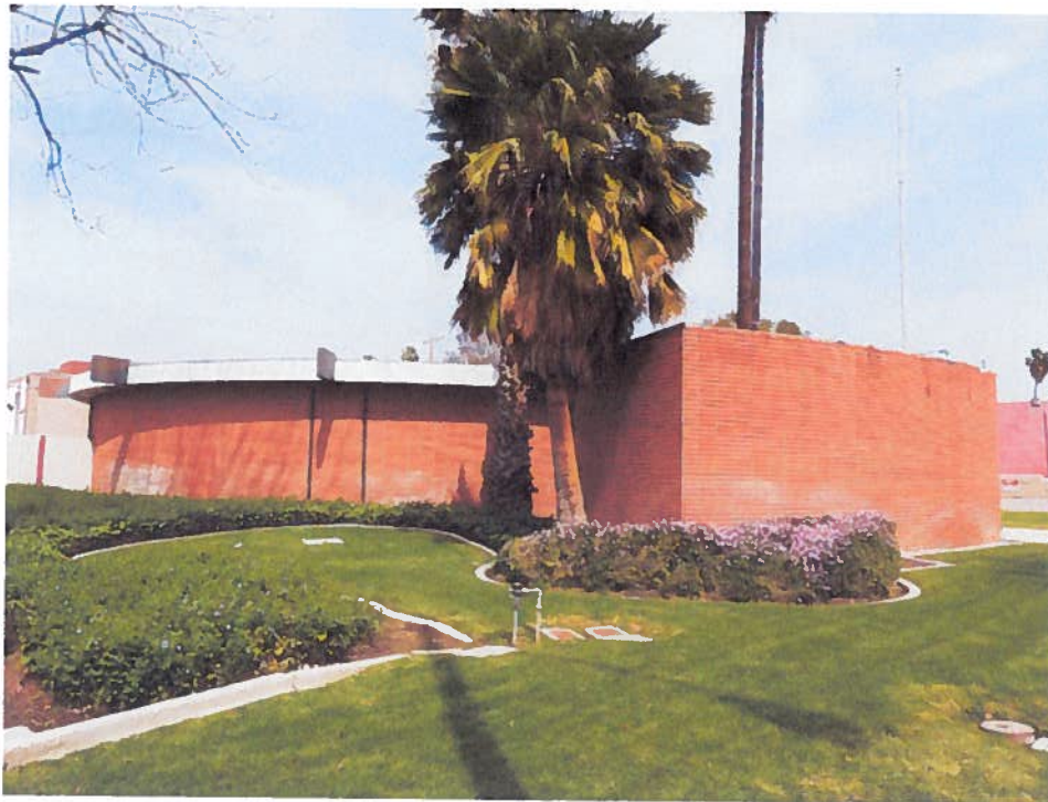
View of West Façade, looking East (March 2013)
