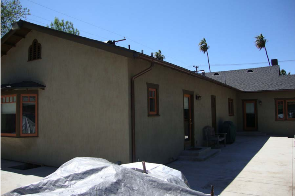
House (Right Side Rear)
