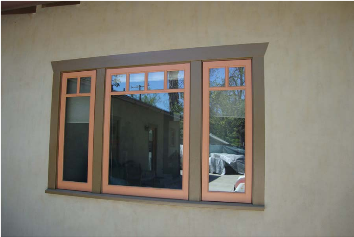
House (Window Detail)
