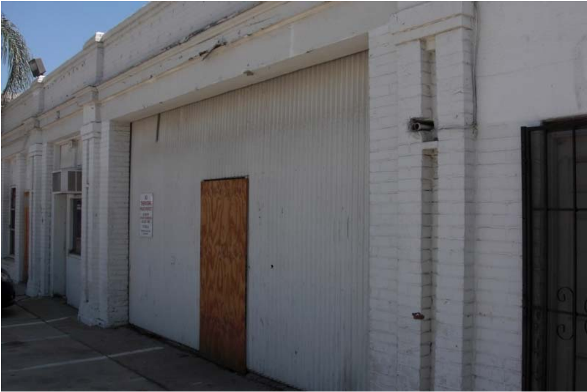
Historic Building (Side Facade Service Bay to be Storefront)
