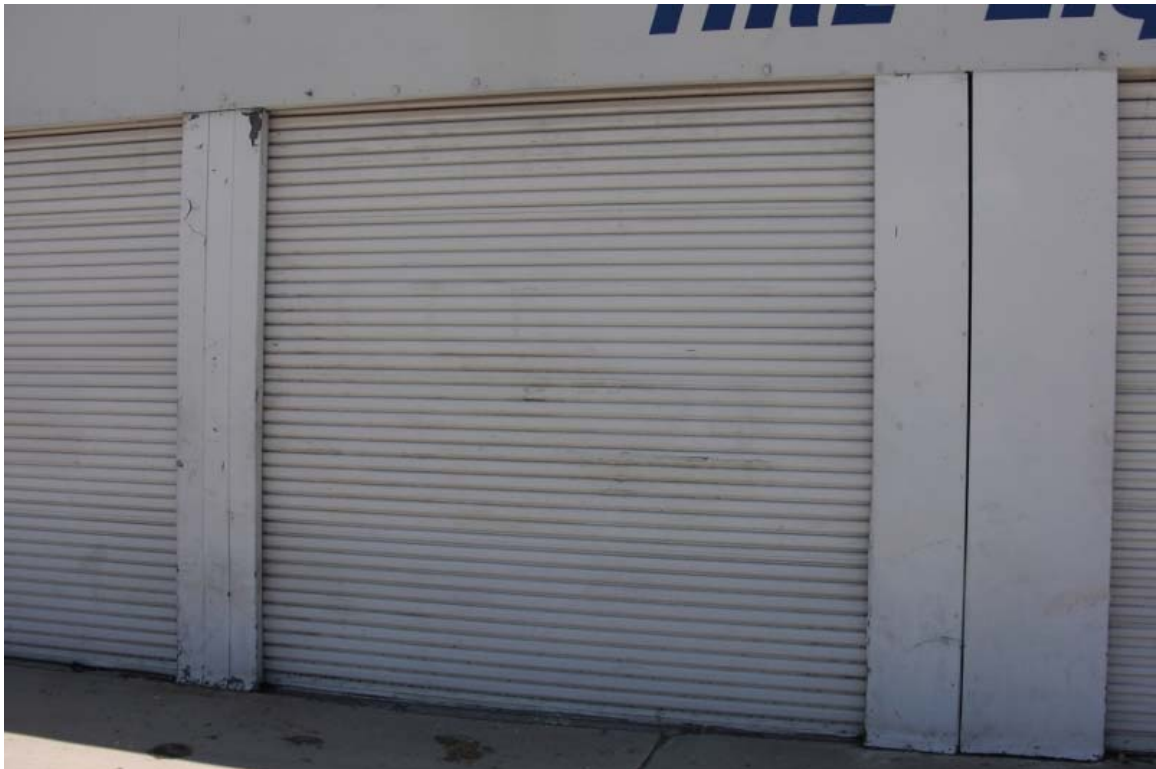
Non-historic Building (Detail of Existing Facade)
