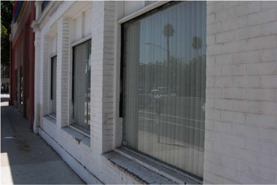
Historic Building (Front Facade Windows)
