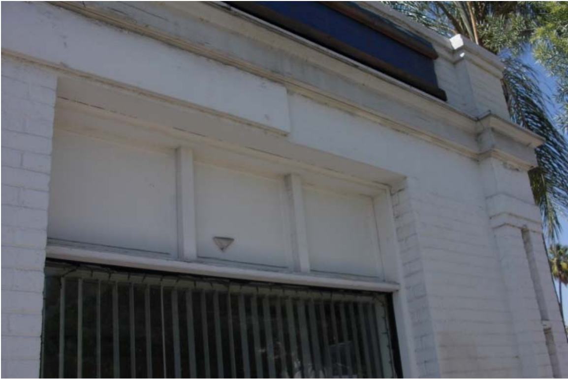
Historic Building (Front Facade Transom Detail)
