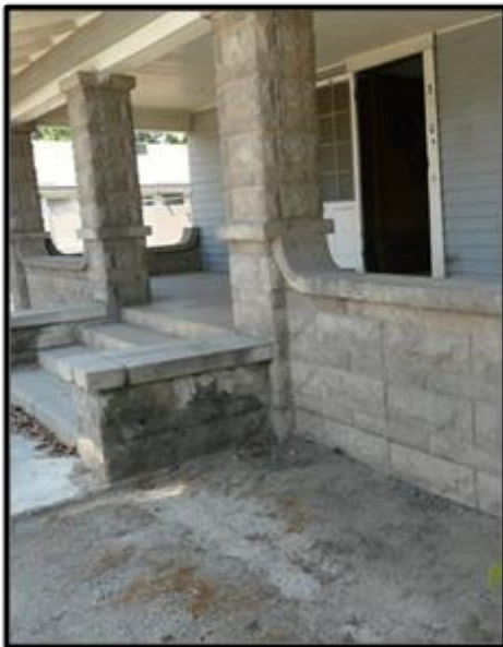
Cooper House details. Clockwise from top left: Deteriorated pot shelf below diamond light window/vent assembly at front gable; full chimney at left side, separating from wall; top of deteriorated wood stairs to attic at rear; pre-cut stone columns and walls at porch with shaped and slab concrete caps.
