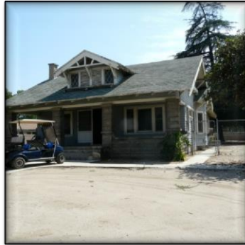
Cooper House front view, 2013
