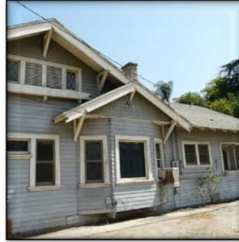
North side, rear portion, 2013
