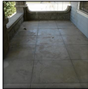
Front porch concrete scoring
