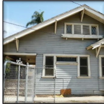
North side, front portion, 2013
