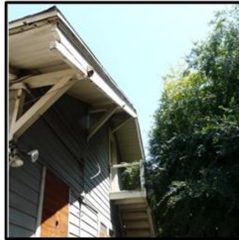
Cooper House details. Clockwise from top left: Deteriorated pot shelf below diamond light window/vent assembly at front gable; full chimney at left side, separating from wall; top of deteriorated wood stairs to attic at rear; pre-cut stone columns and walls at porch with shaped and slab concrete caps.
