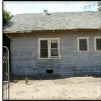
South side, rear portion, 2013
