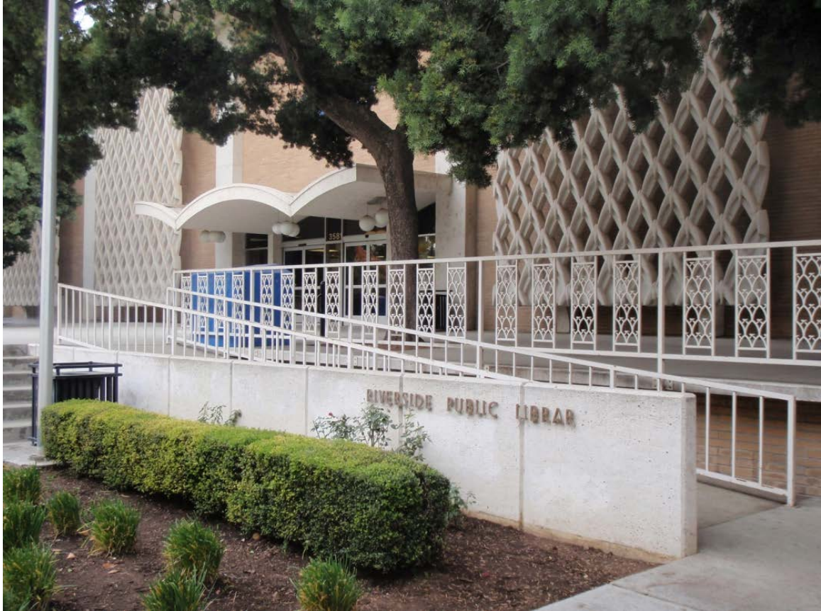
Figure 5 Riverside Main Library, entrance ramp and handrail slated for replacement. Source: Page & Turnbull, December 2011.
