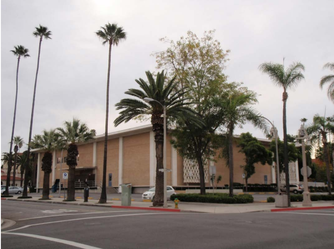
Figure 6 Riverside Main Library, north elevation. Source: Page & Turnbull, December 2011.
