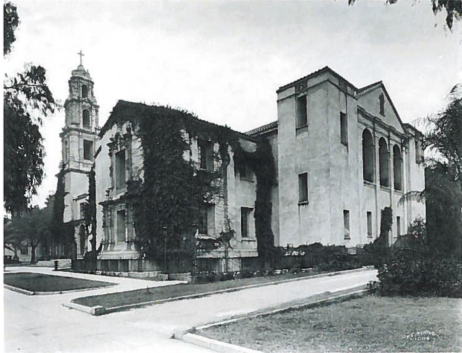
Figure 5 - Historic northwest view from Mission Inn Avenue
