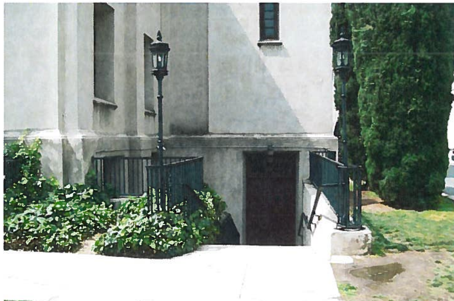
Figure 6 - View into Stair & Patio at NW Corner
