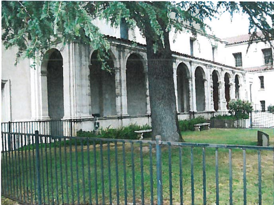
Figure 4 - Close-up View of Loggia
