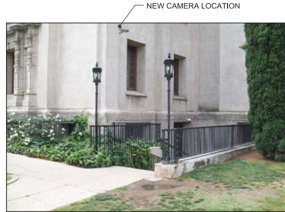
A CAMERA LOCATION AT BASEMENT COURTYARD
