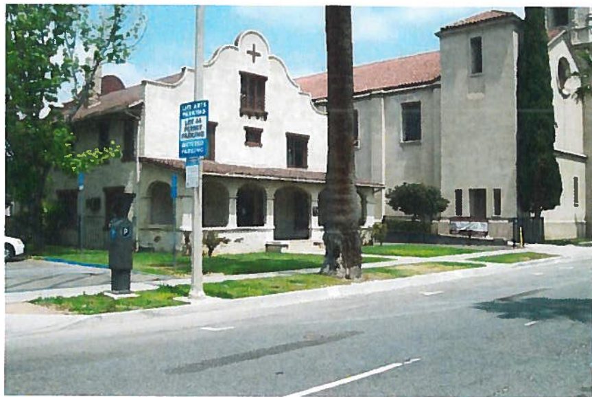
Figure 13 – SE View of Parsonage from Lemon Street
