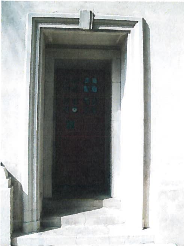
Figure 14 – North Tower Door
