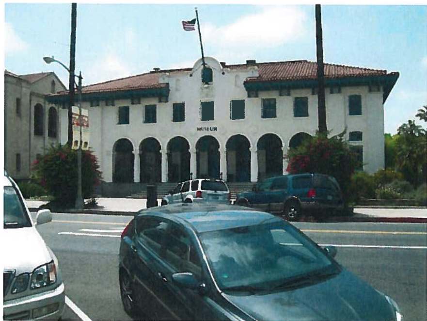
Figure 17 - Grille-Gate in Entry of Riverside Municipal Museum
