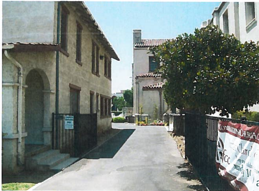
Figure 11 - Driveway between the Parsonage & Church
