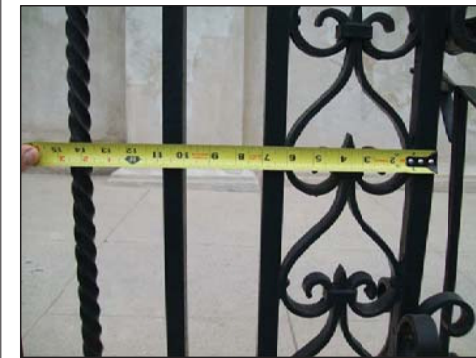
TYPICAL HISTORIC HANDRAIL-MEASURED
