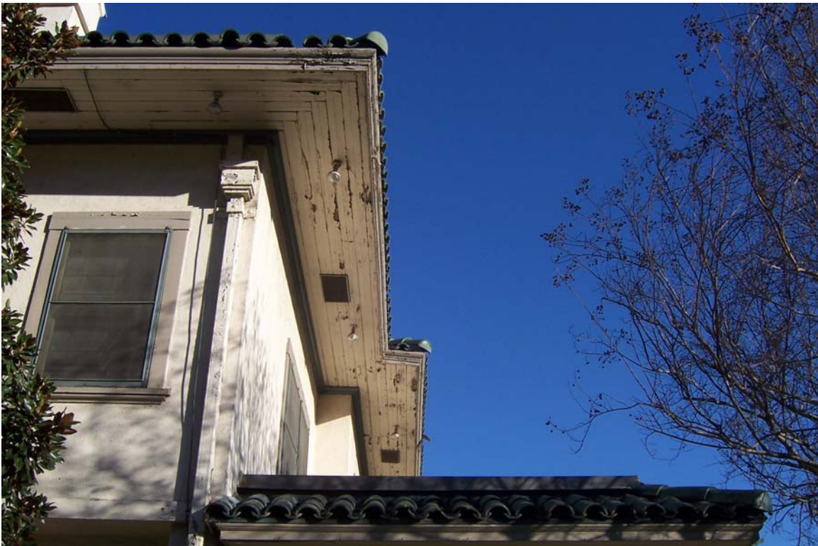
P11-0795, Exhibit 3 Site Photos
