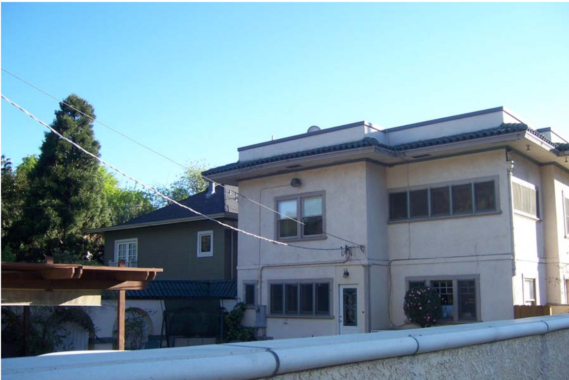
P11-0795, Exhibit 3 Site Photos
