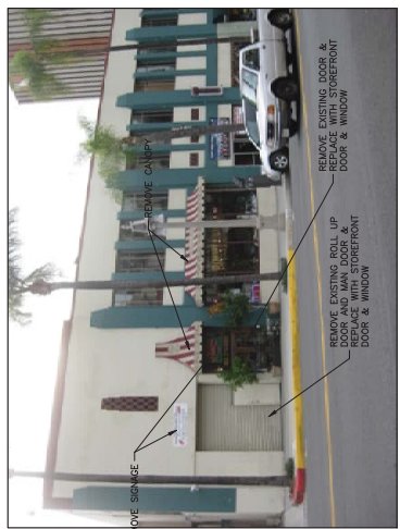
NEW STORE FRONT SYSTEM LOCATION NO SCALE
