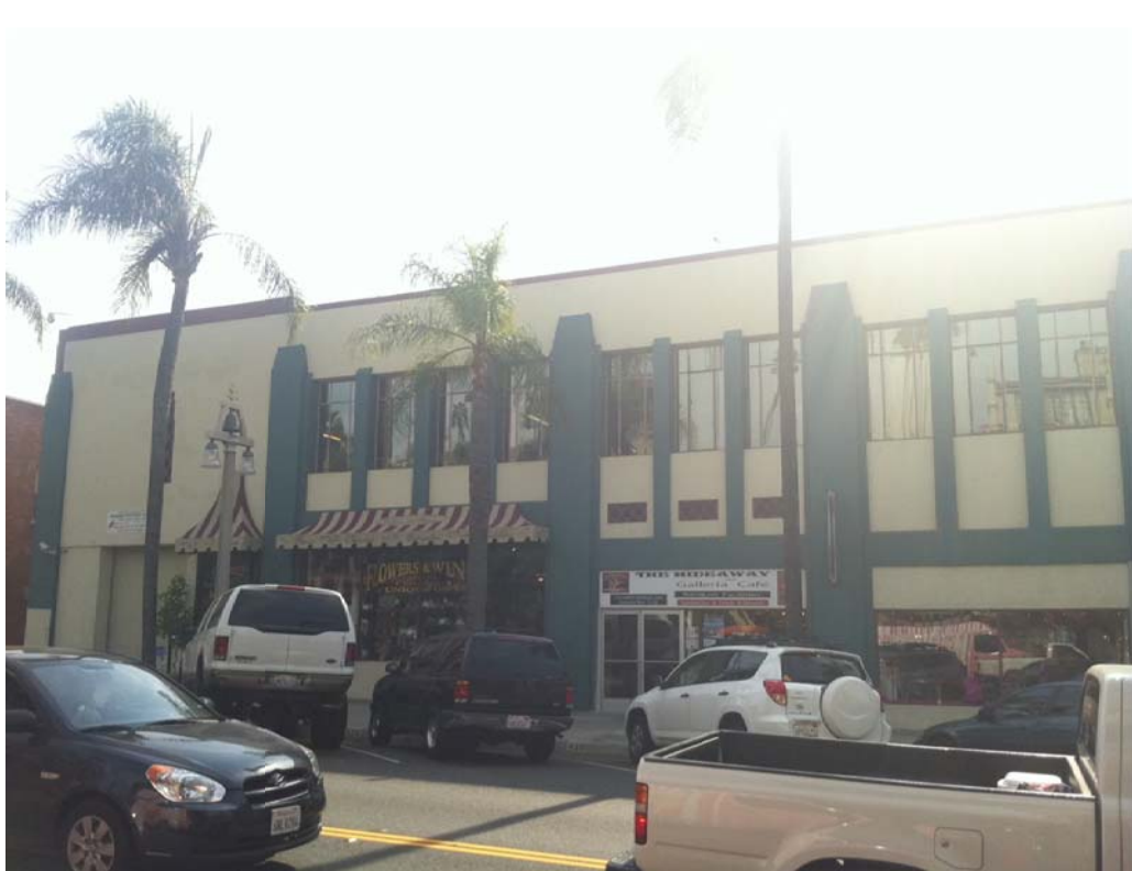
P11-0138, Exhibit 6 Site Photos
