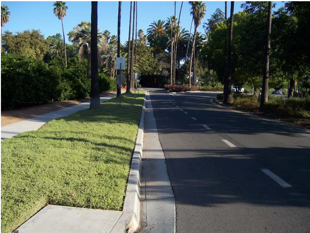
Existing Victoria Avenue frontage
