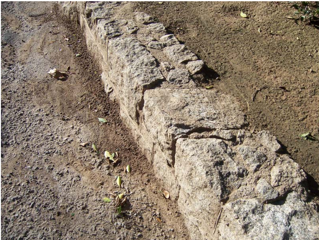
Existing low rock wall
