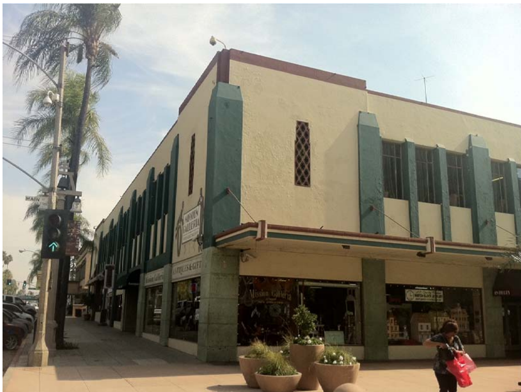
P11-0138, Exhibit 6 Site Photos
