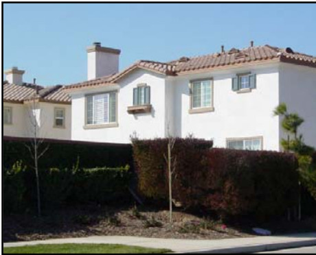
Multi-paned windows are treated with decorative moldings, exposed dentils, decorative shutters and window planter boxes. See guideline III.A.3.h.
