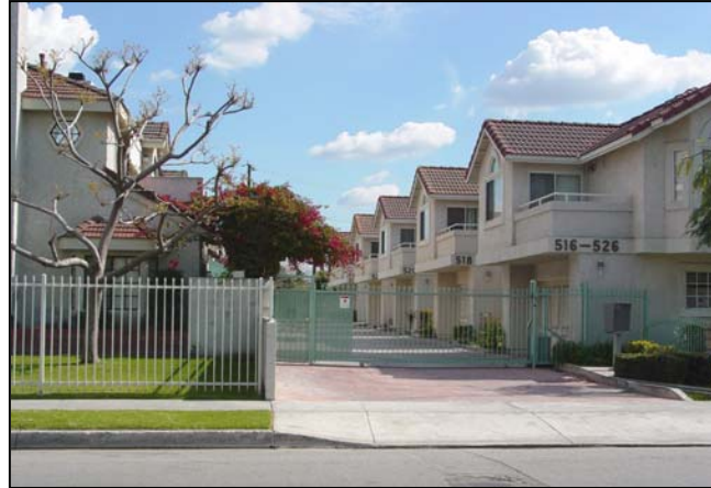
Avoid siting dwellings where vehicular and pedestrian access are together. Keep pedestrian and vehicular access separate.
