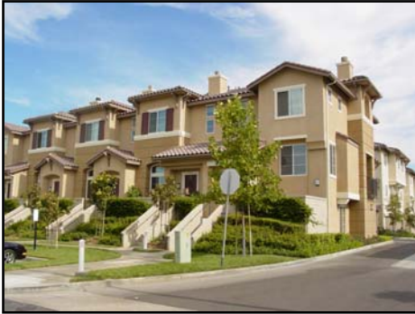
First floor level is raised for privacy and security. See guideline III.B.4.c.
