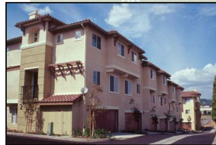
Rear landscaping softens stark appearance of garage doors on alley-loaded development.
