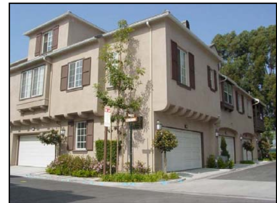
Garages are integrated architecturally with the structure so that they are not a dominant feature. See guideline III.B.3.b.
