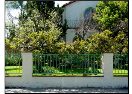
Front yard fencing and walls such as low garden walls and wood pickets or wrought iron should provide the appearance of visual openness. Use landscaping such as clinging and climbing vines to soften their appearance while still maintaining this openness. See guideline III.A.5.b.
