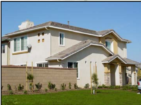
Rear and side elevations are treated with the same high-quality details as the front of the house. See guideline III.A.3.i.
