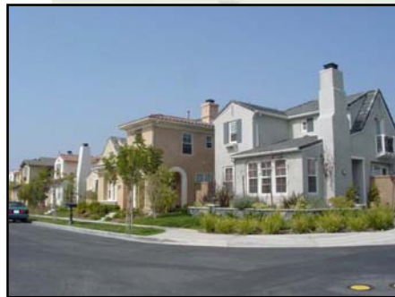
Attractive streetscape is achieved with compatible scale and massing between structures. See guideline III.A.7.b.iii.
