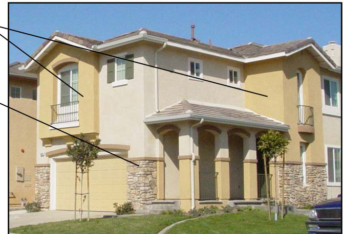
Natural stone is used consistently around all major wall planes of the home at the first floor only and covering more than three quarters of the first floor level providing the appearance of a natural foundation. Trim is used to finish the appearance of the faux exposed stone foundation in a cost-effective and highly attractive manner
