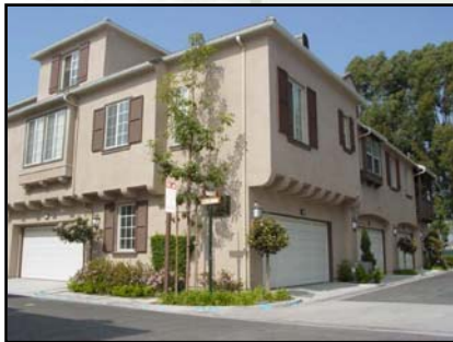
Rear and side façades are finished consistent to the front. See guideline III.B.4.i.
