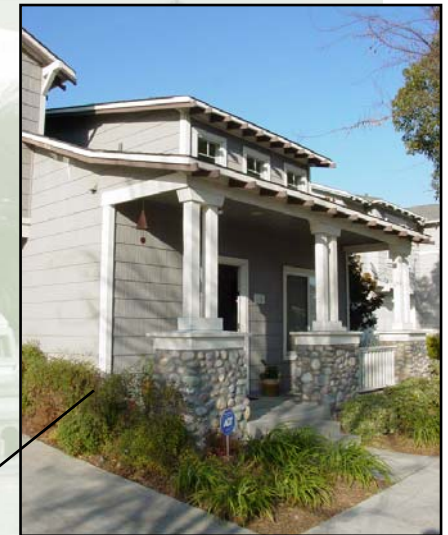
Utilities screened from public view behind landscape hedge
