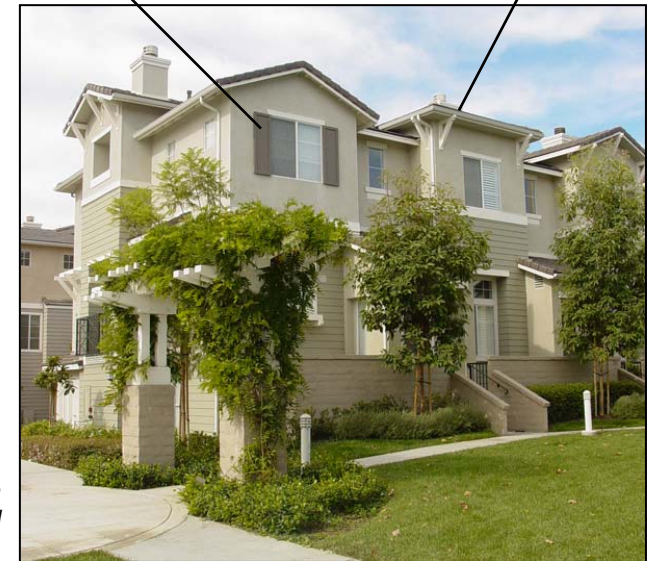
High-quality design elements for multi-family buildings can include window shutters, exposed rafter tails, vine-covered trellis, and different building façade materials.
