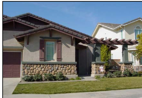
Architectural details on these new Craftsman style homes such as front porches, wood columns, exposed rafter tails, and fascia provide a high quality appearance.
