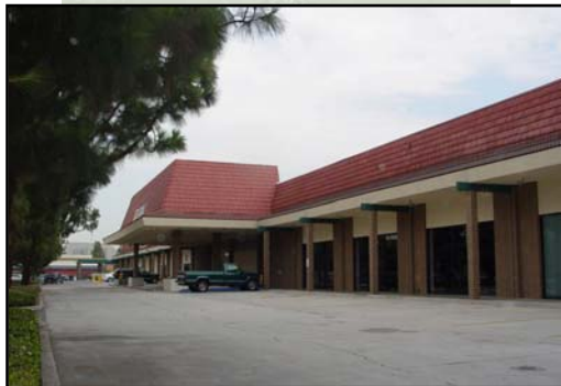
Vacant older neighborhood shopping center with dated appearance
