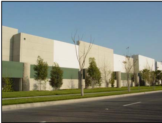
Treatment of this industrial building's well-articulated façade is encouraged.
