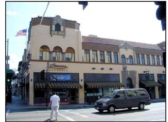
High quality architecture can create a highly stylized building. See guideline IV.D.3.C.1.
