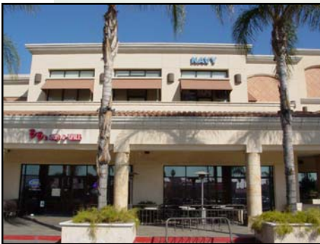
The setback of the second story avoids a monotonous façade. See guideline IV.D.3.B.1.
