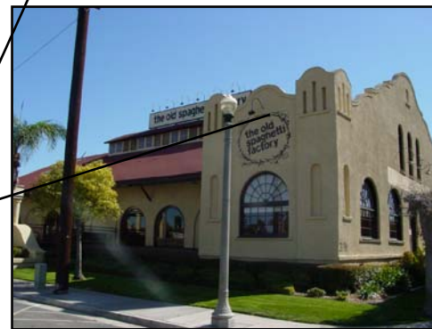
Parapet walls in the classic mission shape
