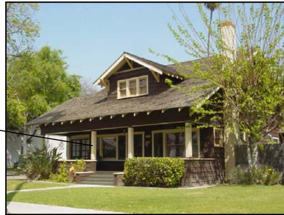
Exposed rafter tails Low-pitched roofs Unenclosed eave overhangs
