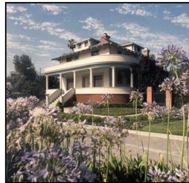
Prominent porch with rounded columns
