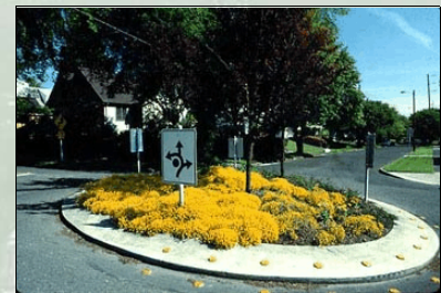
Traffic-calming features include small roundabouts like this one that reduce the speed of neighborhood traffic and enhance the neighborhood's appearance.
